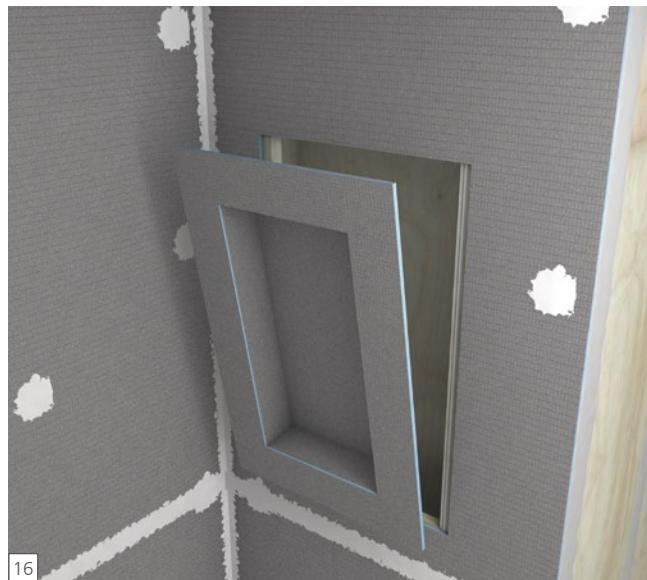
**EN** 2 Fasteners each side of the niche are set to create a flush transition to the wall panels. Another 1/2" (12.7 mm) bead of wedi Joint Sealant is spread over fasteners and seams.
